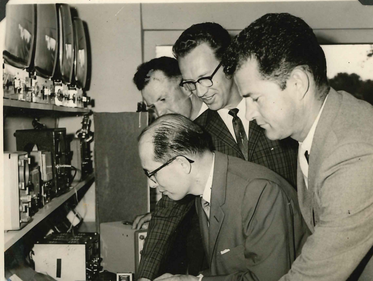
BOB HAMILTON DEMONSTRATES ELECTRICAL ASSEMBLY ON A "BREADBOARD"
