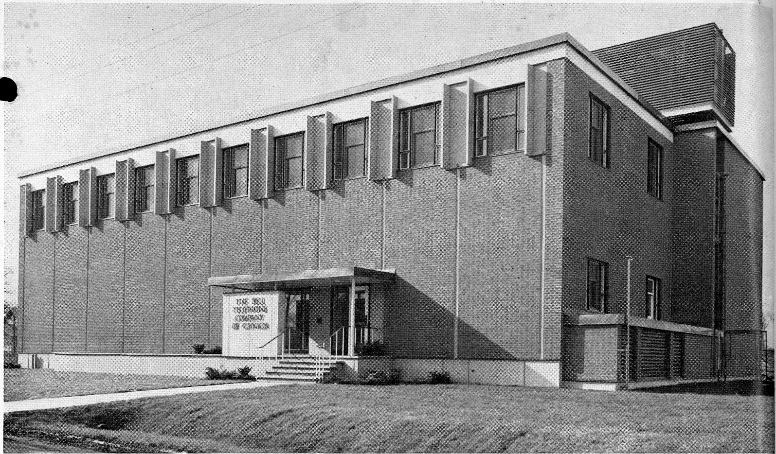
FORT ERIE'S NEW DIAL EXCHANGE BUILDING
