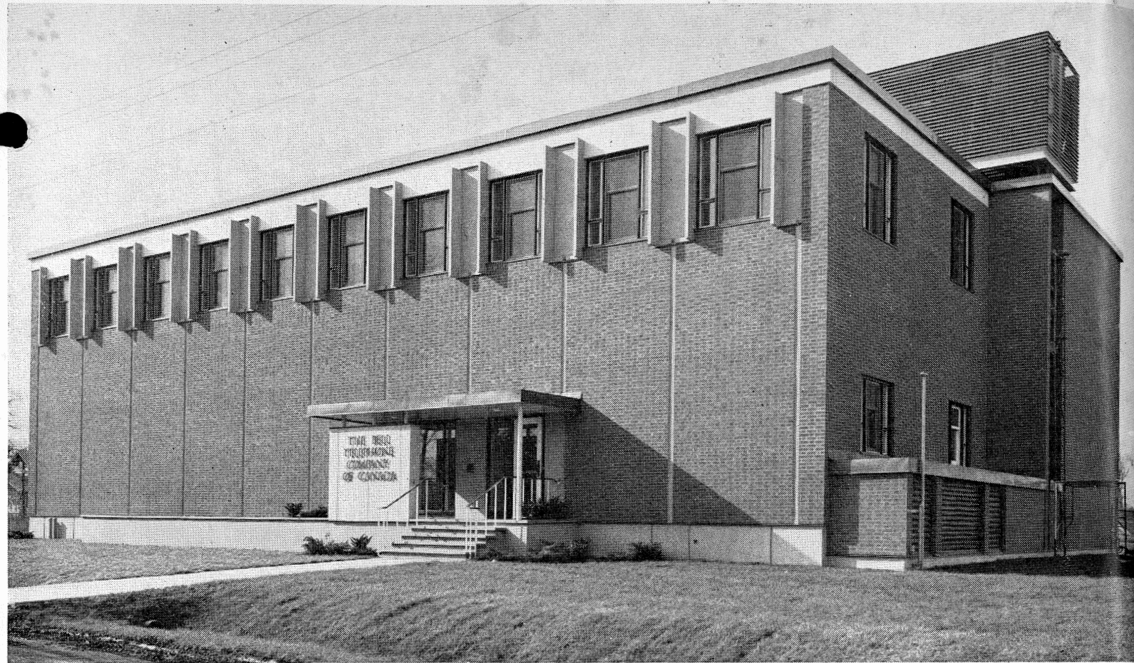
FORT ERIE'S NEW DIAL EXCHANGE BUILDING
