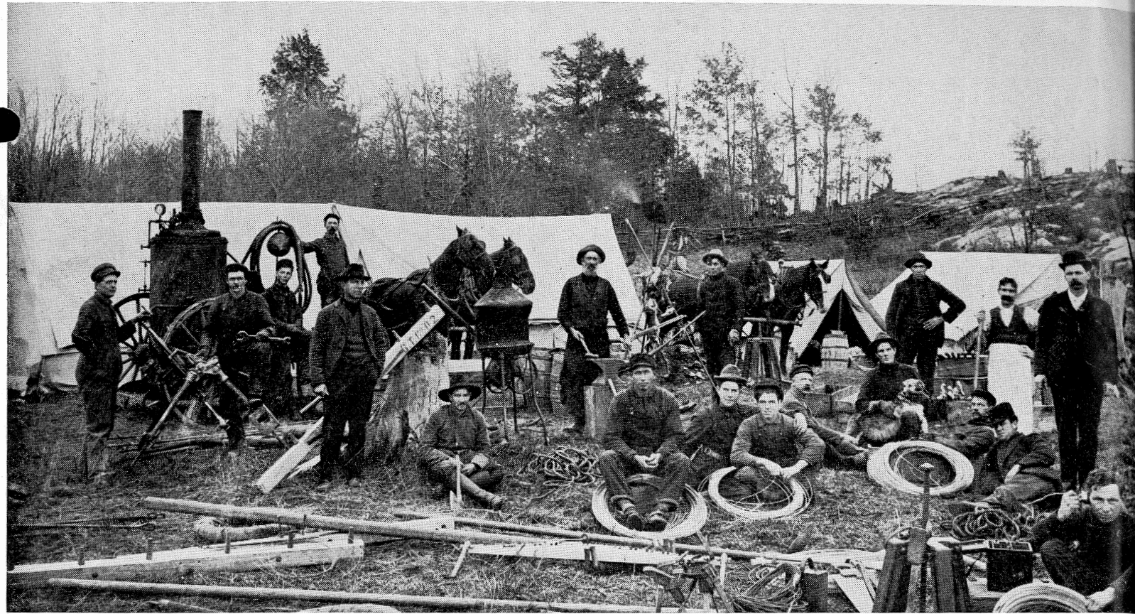
THIS CONSTRUCTION CREW of the early 1900's posed for the cameraman at the end of a hard day's work. The bearded blacksmith and mustachioed cook were essential members of the team. The horse drawn steam boiler was used to provide power for pumping and
